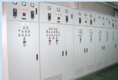
After the adjustment of air-conditioner (cabinet energy-saving inverter was installed)
