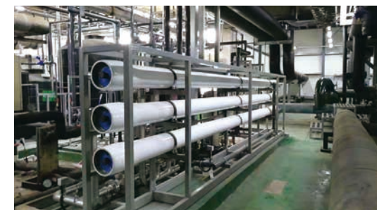
Jigsaw process water reuse system (Zhangjiang Facility)
