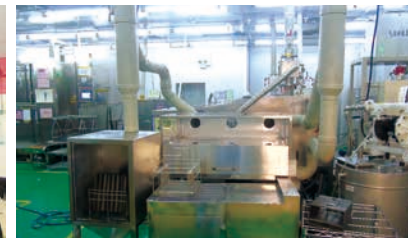
Leigang Cleaning Machine after having Installed Exhaust System (Jinqiao facility)
